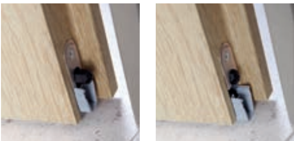
Standard features in sound protection doors: mechanical ground seal
